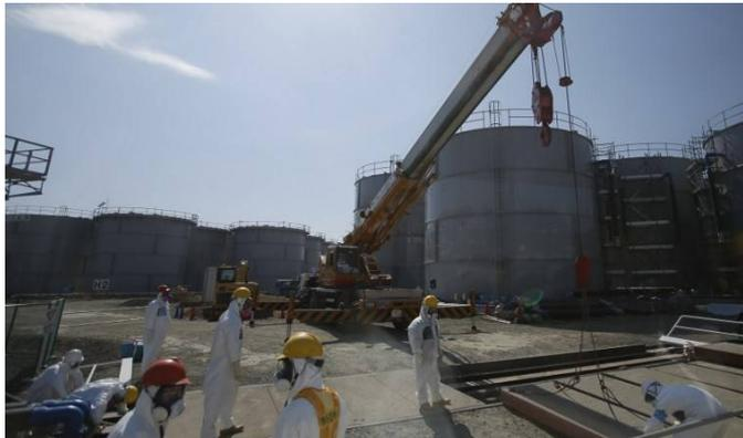
Secondly, setting-up of a new multi-nuclide removal equipment called ALPS, and of pools to store treated water
